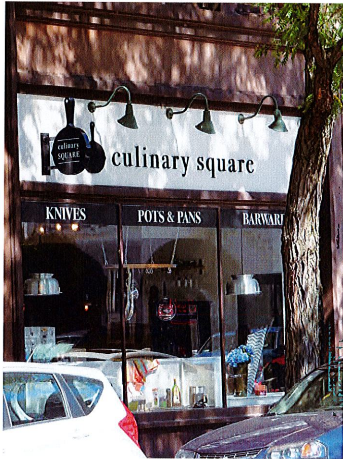
Gooseneck lighting is used to illuminate a wall sign.
